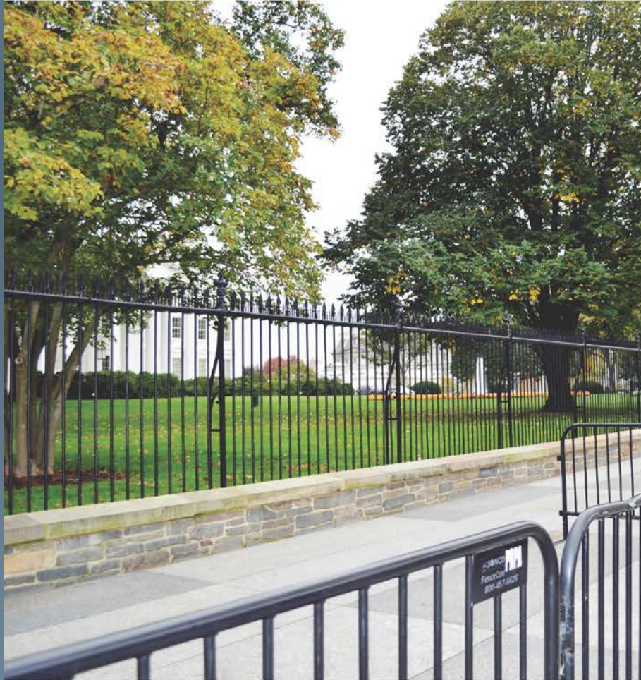
North side along Pennsylvania Avenue Existing Conditions
