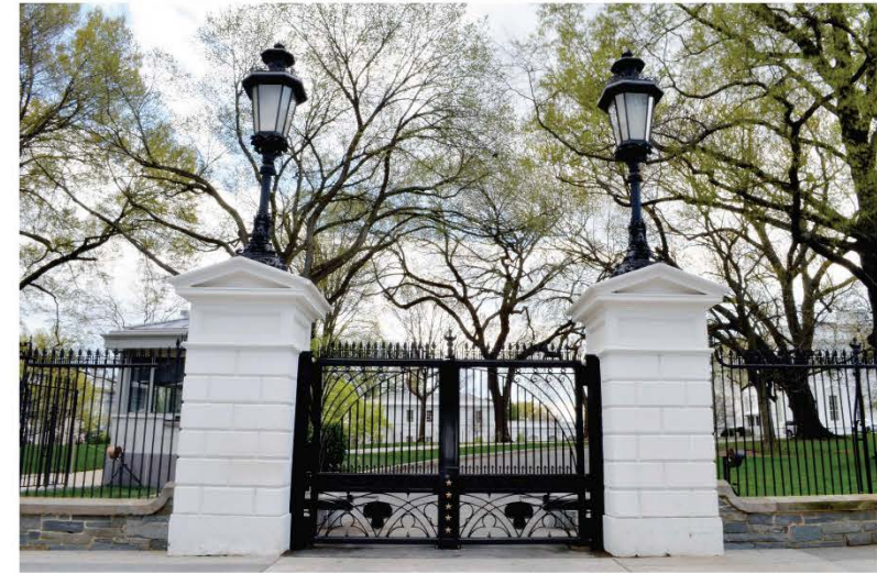
Vehicle Gate Gate to circular drive from Pennsylvania Ave
